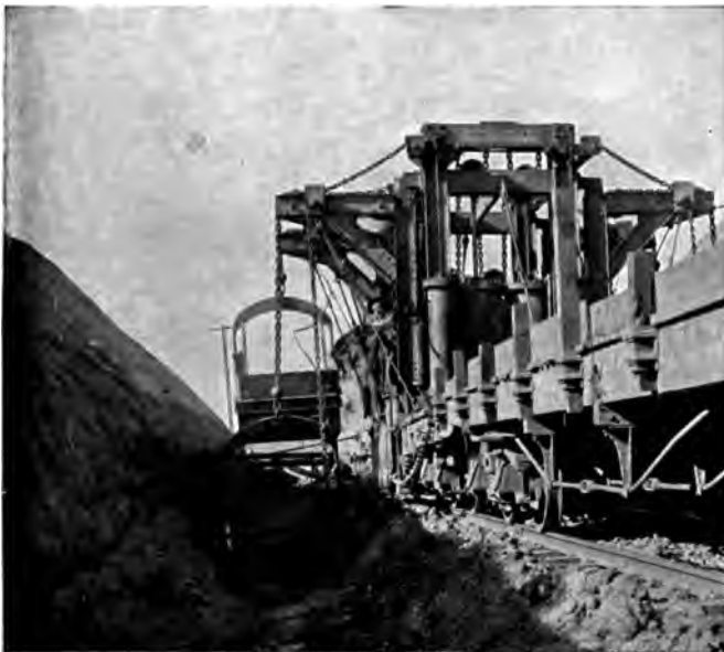
Loading Material into Buckets
